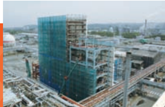
Anode Materials Plant (under construction)
