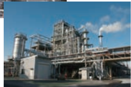
PPS plant at Iwaki Factory
