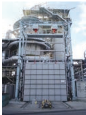
Facility to detoxify low-concentration PCB wastes [Kureha Ecology Management Co.]
