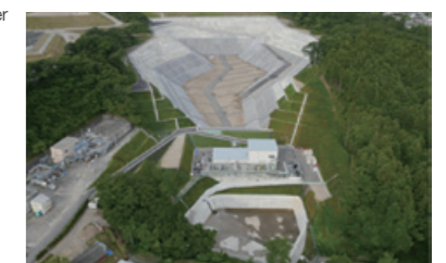
Himeyuri Sogyo Co., Ltd. (Industrial waste final disposal plant)
