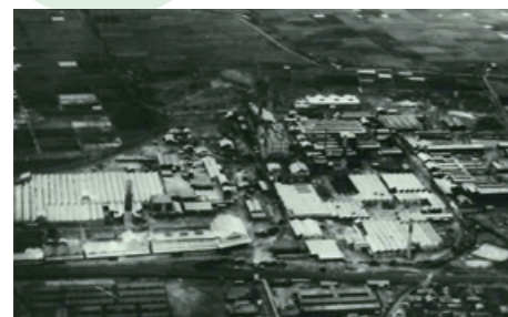
Kureha Chemical Industry Nishiki Plant
