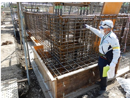
In-house inspection of a building's foundation
