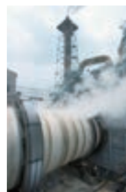
Industrial waste treatment facility
