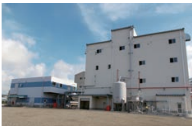
PVDF production facility at Iwaki Factory
